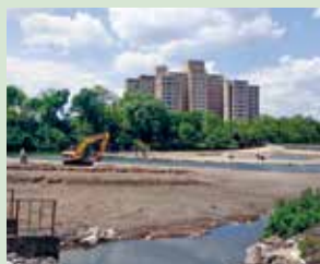
Placing clean sand for plants
