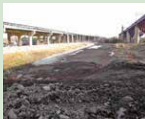
During site excavation
